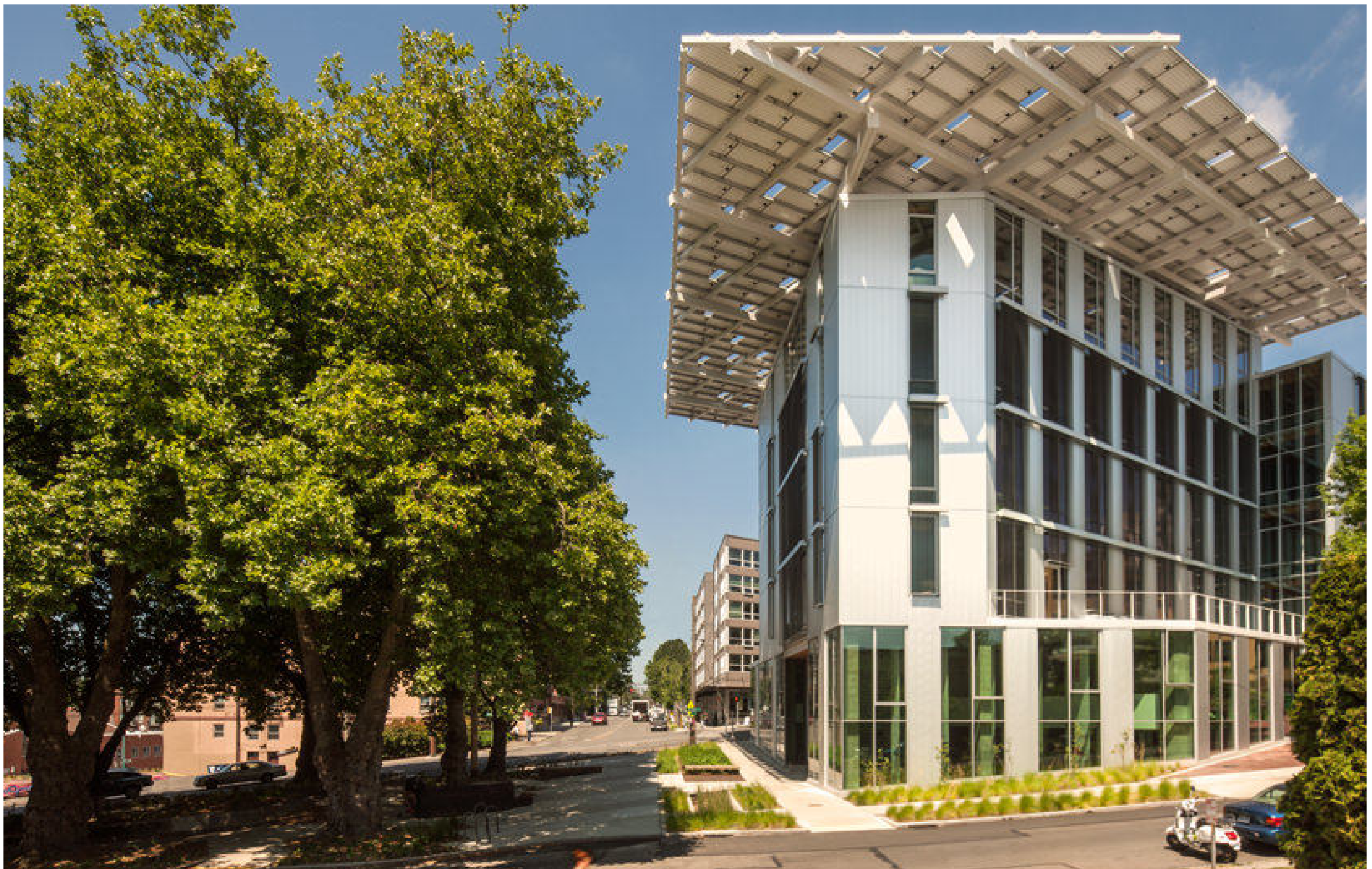
Image source: Bullitt Center
